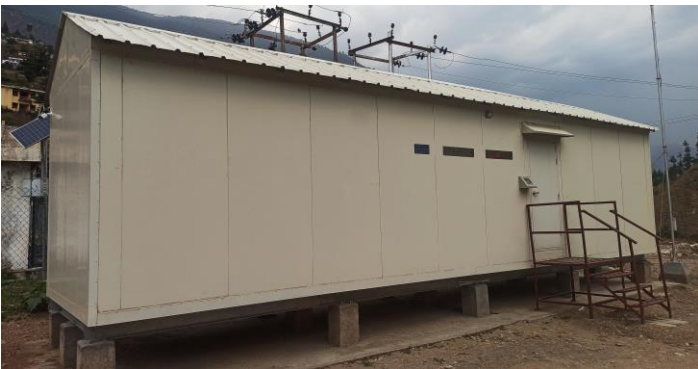
Command & Control Centre
