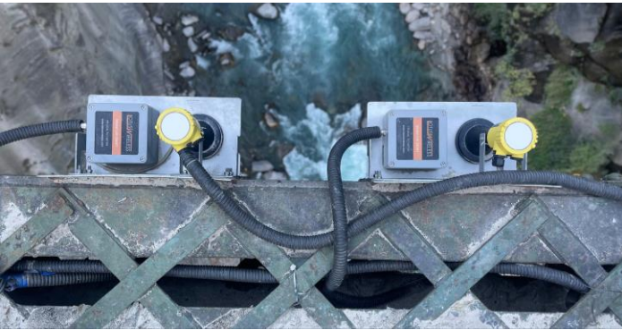
Sensors Position on Bridge
